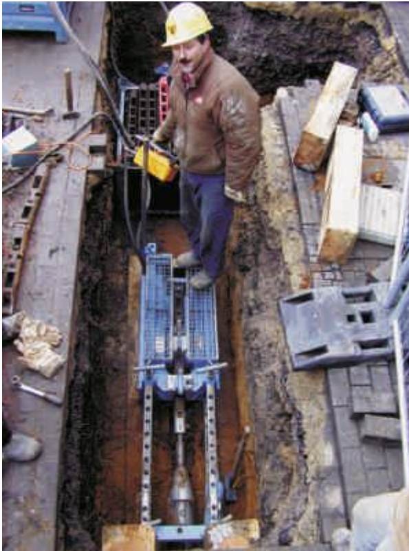
Fig. 1.10: Static Pipe Bursting
