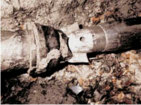
Fig. 1.5: Grundocrack bursting blade destroying a pipe joint
