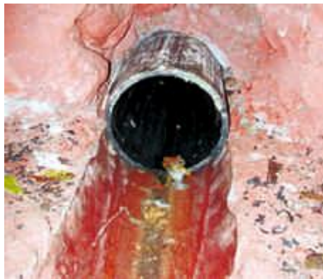
Fig. 1.11: PE-pipe installed with calibre bursting
